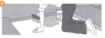
Fold back both edges by half the width of the carpet taking care not to disturb the positioning of the carpet. Apply the recommended adhesive to the subfloor using the application technique recommended by the manufacturer, then re-position the first piece of carpet and roll with a 68kg flooring roller to ensure overall contact with the adhesive.
