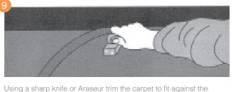
Using a sharp knife or Araseur frim the carpet to fit against the perimeter walls.
